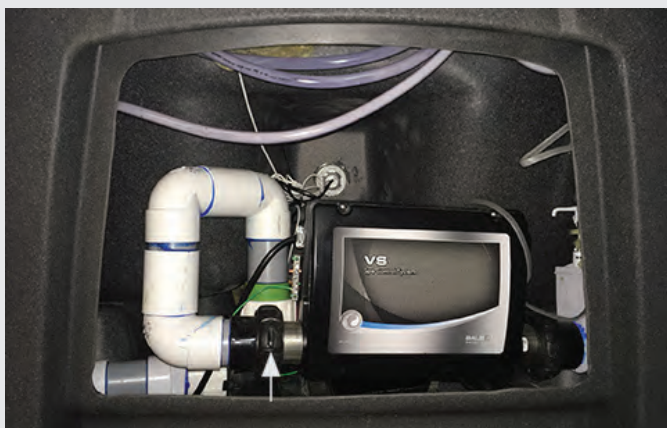
FIGURE 1.9a : HEATER UNION; LOOSEN UP TO BLEED AIR
